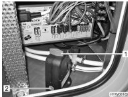
Fig. 92 Safety/drainage valve of the boiler
